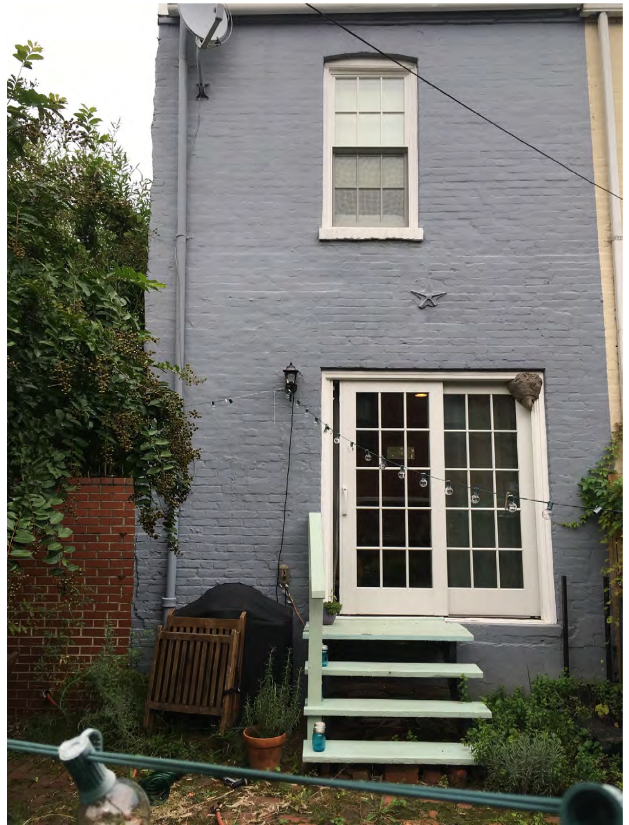
EXISTING REAR FACADE
